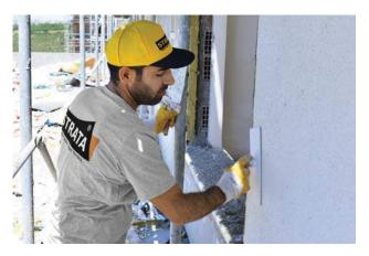
It is a white cement based, polymer-added, mineralized textured, waterproofing top coat decorative facade coating offering an aesthetic appearance thanks to its special filler dimensions and it is applied as final coat before paint.
