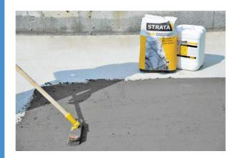
MS - 09 which forms a waterproof insulation layer when applied by spreading is a polymer based, single component water insulation product.
