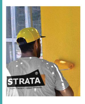
Silicone emulsion based, exterior top finish applied with a roller and textured with roller.
