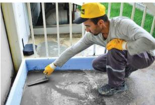
Cement based, polymer-reinforced, gray colored leveling mortar in powder form composed of environmentally friendly additives; has a fluid structure, self-leveling floors and a high performance in removing surface irregularities; ready to use in a short time.
