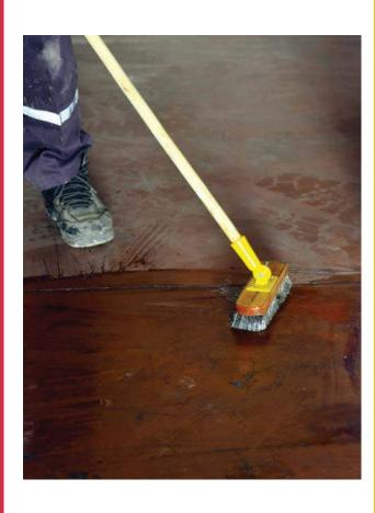
It is a cement-based, polymer-reinforced, environmentally friendly rectifying screed, ready to use in a short time with a fluid structure, by fast freezing and at an average thickness of 10 cm.
