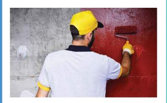
POLIWHITE is a waterproofing material that is applied in liquid form and has very superior properties, which, when dried, turn into flexibilty, impermeable, solid coating.
