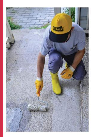
It is an acrylic resin-based curing material applied on concrete, screed and cement based surface hardener, forming a protective film layer that does not penetrate water vapor and prevents cracking on the surface.
