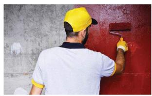
POLIKIT is a one component, plastic, glossy coating and flexible waterproofing material based on acrylic elastomeric resin which is applied by spreading.
