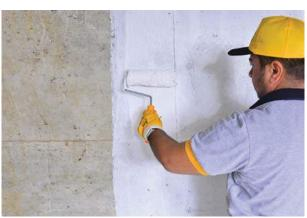
POLITIGHT is a one component, plastic, glossy coating and flexible waterproofing material based on acrylic elastomeric resin applied by spreading.
