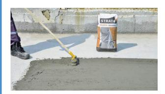
FW 2K is a high quality semi-flexible waterproofing material that continuously protects the two-component flexibility of cement and acrylic-based powder and liquid binder.
