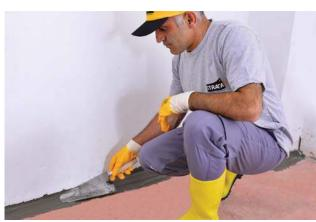
It is a cement based, non-shrinking, self-spreading anchorage and repair mortar with high adherence and strength.
