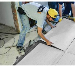
TILEBOND FLEX is a cement-based, polymer-added single component, environmentally friendly C2T class tile size ceramic marble and granite bonding mortar developed in TSE Standards which has ultra strength and enhanced adhesion, reduced slip, facilitated workmanship through longer working time.
