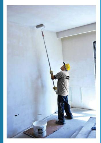
Polymer modified resin based interior and exterior surface primer that will be used to increase surface adherence before gypsum and cement based mortar applications on fair faced finish concrete.
