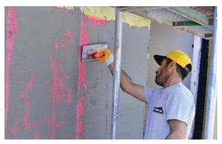
It is a white cement based, polymer additive mineralized textured waterproofing top coat decorative facade coating with special filler dimensions that offers an aesthetic appearance and applied as final coat before paint.
