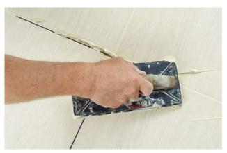
FLEX FUGA JOINT is a joint filling mortar with various color options which is reinforced with polymer additives, contains silicone and white cement-based, polymer-compounded for using at joint formations between glazed tile, ceramic, mosaic, marble, granite and similar tiles and conforming to TSE standards, easy to apply and forms a smooth surface, and applicable at 1-6 mm thickness.
